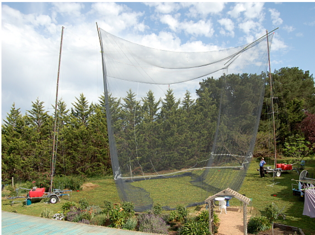
Fig 10: Enclosure net mounted between the assembled masts. Pic by Daryl King.
